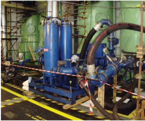
A flushing skid in operation
