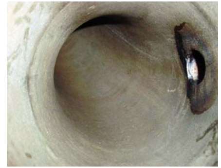
An oil pipeline after hydroblasting
