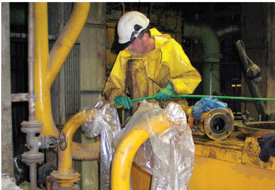
Hydroblasting of an oil system
