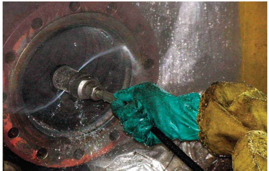
The hydroblasting process
