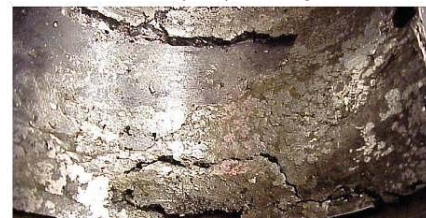
FIGURE 5. Loss of overlay (Babbitt) material down to the base metal
