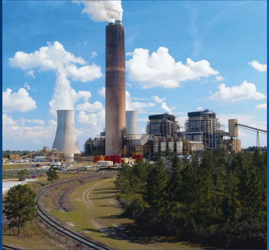
After switching to condition-based oil changes, the Seminole Electric plant was able to achieve a cost avoidance of $1.27 million over a five-year period.
