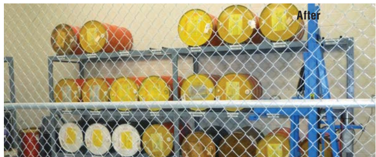
The first-in/first-out method is now used for storing oil drums.
