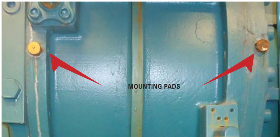
Installing brass pads in mounting locations allowed for repeatable data collection.
