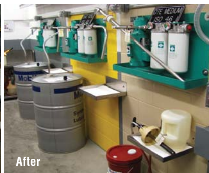
Each type of oil has a separate pump and filter system to filter and fill the portable containers. The bulk systems in the field and the filter carts are equipped with identical pumps and filters. Recirculation lines to circulate oil in the drums are planned for the near future.
