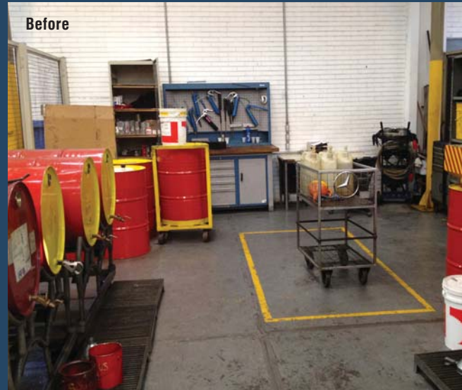
The previous lube room had several sources of oil contamination.
