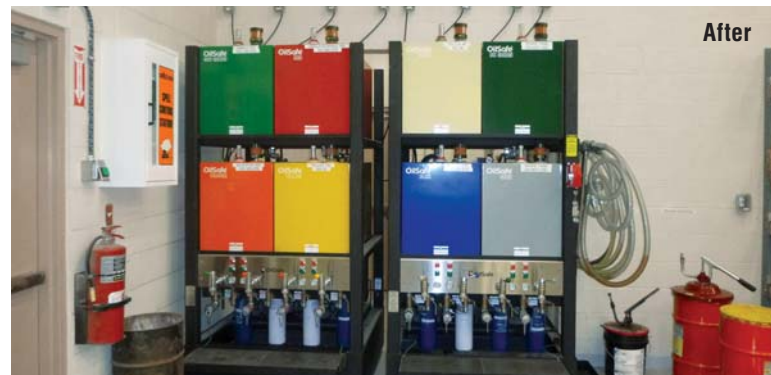
Now all oil is filtered at least twice and sometimes three times.
