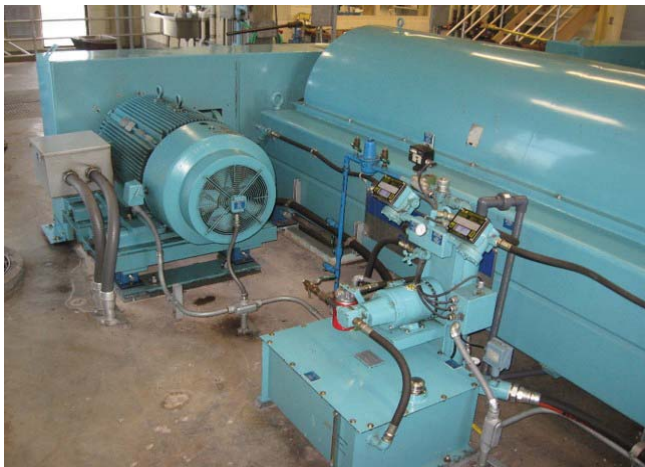
A 300-horsepower, AC-induction motor and bowl drive assembly
