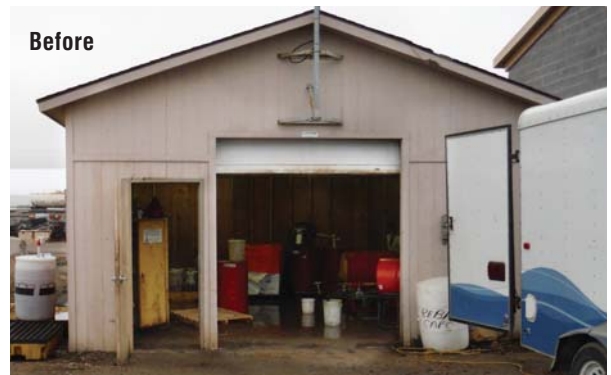
Compass Minerals' old lube building was not secure or organized.
