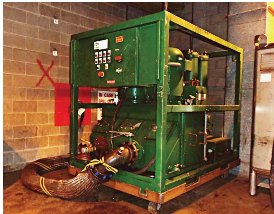
A large pump/filtration unit provided the circulation for the system flush.
