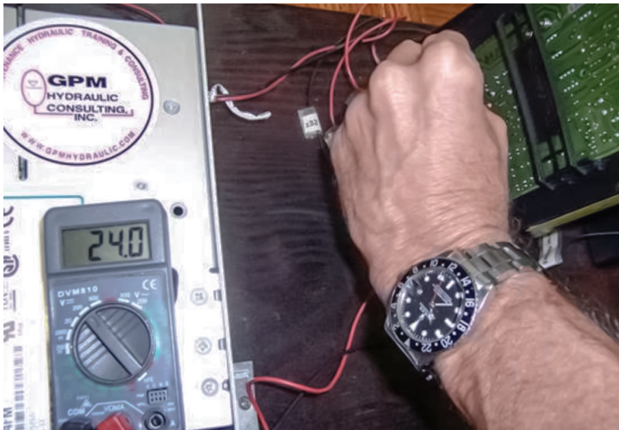
Figure 7. A good power supply is indicated by 24 volts at the amplifier.
