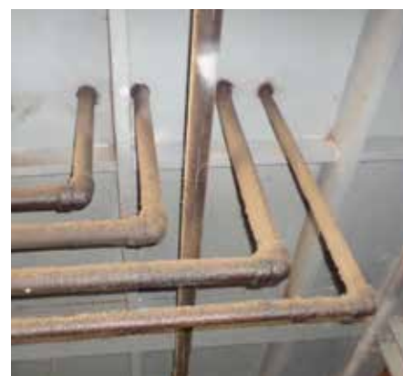
The use of 90-degree fittings in the pipe and tubing should be avoided when plumbing a system.
