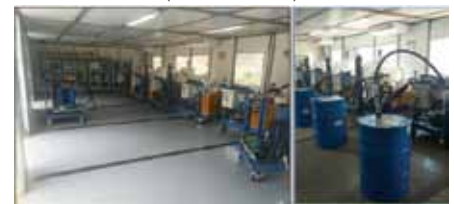
An internal view of the plant's lubrication workshop
