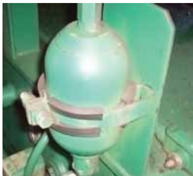
Figure 1. A bladder accumulator
