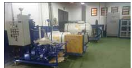
The pipeline lubrication workshop
