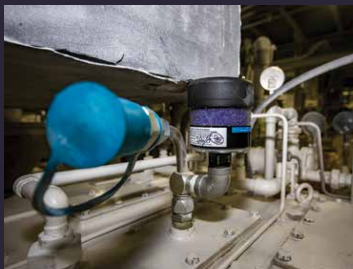
The drain mount (left) and breather mount (right) installed on a vital piece of equipment
