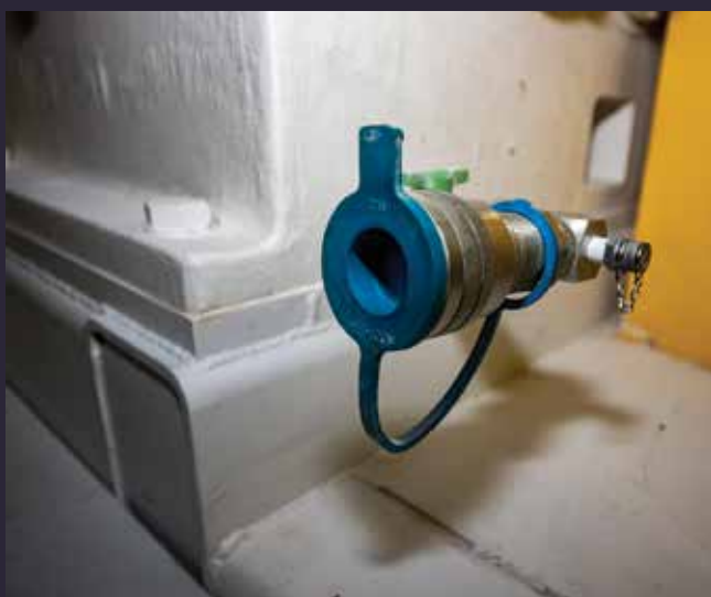
The drain mount (left) and breather mount (right) installed on a vital piece of equipment
