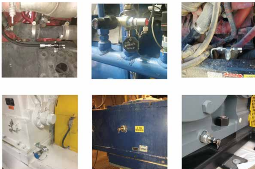
Figure 3: Examples of Dedicated Sampling Valves
