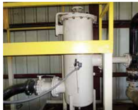
Kidney-loop system filters may be quite large.
