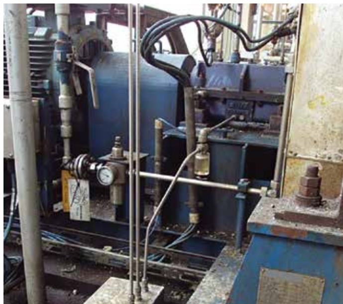
Figure 4. A gas blower lubricated by oil mist.
