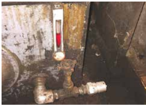
Figure 2. Use protective covers and wipe down quick connect fittings before attaching any equipment.
