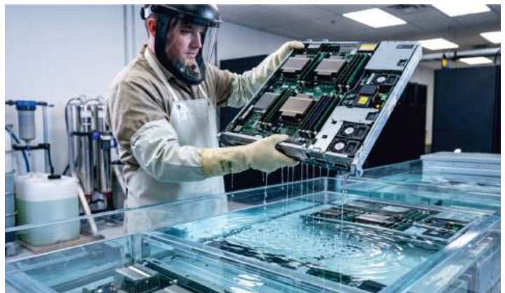
Hardware removal from an immersion tank demands full PPE and accounts for fluid carryout losses.
