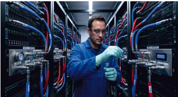
Routine coolant sampling on a live direct-to-chip loop.
