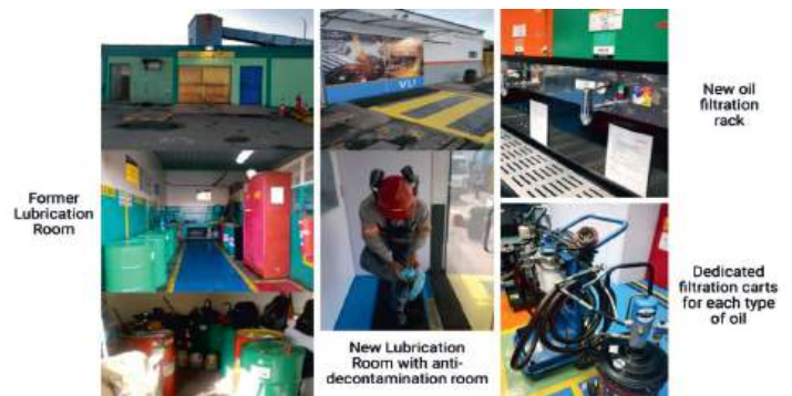
Before and After: Lubrication Room
